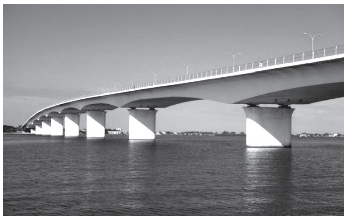
Rys. 6. Most Ringling Causeway (Jeff Pouliotte: PT Grouting and Corrosion Issues in Florida)
